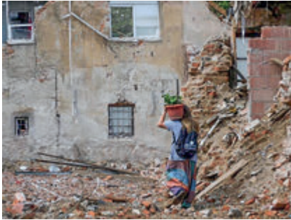
Fig. 1. The city of Petrinja, Croatia, ravaged in the wake of an earthquake in December 2020. The region was first left in ruins by the 1991–1995 Croatian War of Independence and had not recovered.
